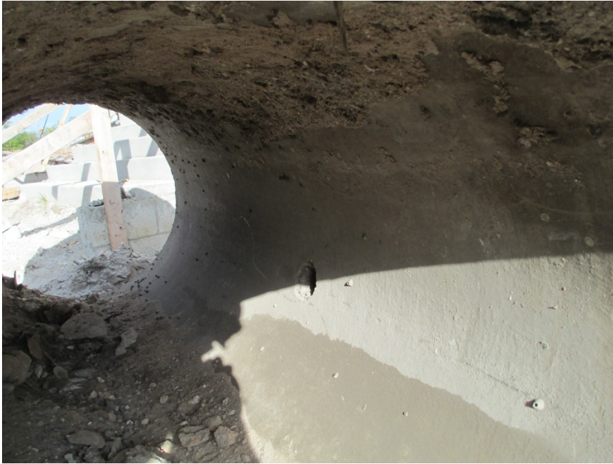
Figure 4. A lift hole, cored into the pipe at casting, is visible in the 30-year old steel reinforced concrete pipe removed from the Dania Beach marina renovation. Although installed at an outfall in a tidal seawater environment, there is no visible deterioration adjacent to the lift hole.
