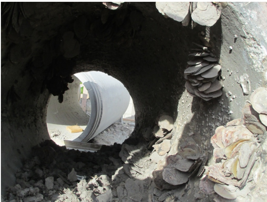
Figure 1. Barnacles attached to the inside barrel of concrete pipe after 30-years in the tidal Dania Beach marina.
