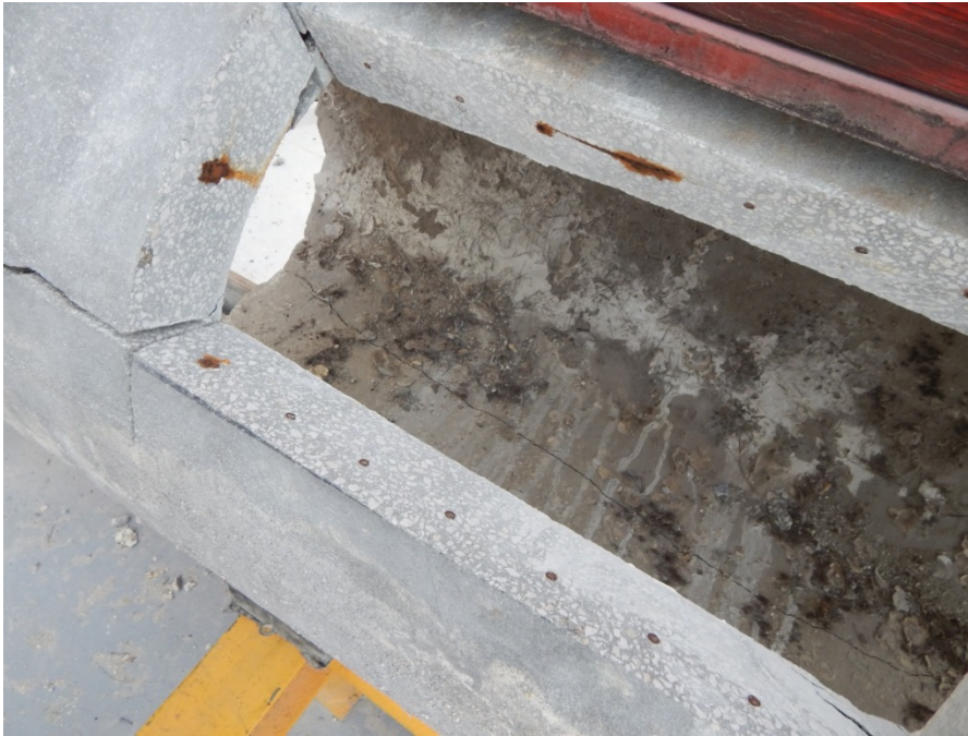
Figure 2. A 1-foot by 2-foot section was cut from the barrel to observe and measure steel reinforcement. Minor steel corrosion was observed, but with no damage to the adjacent concrete.
